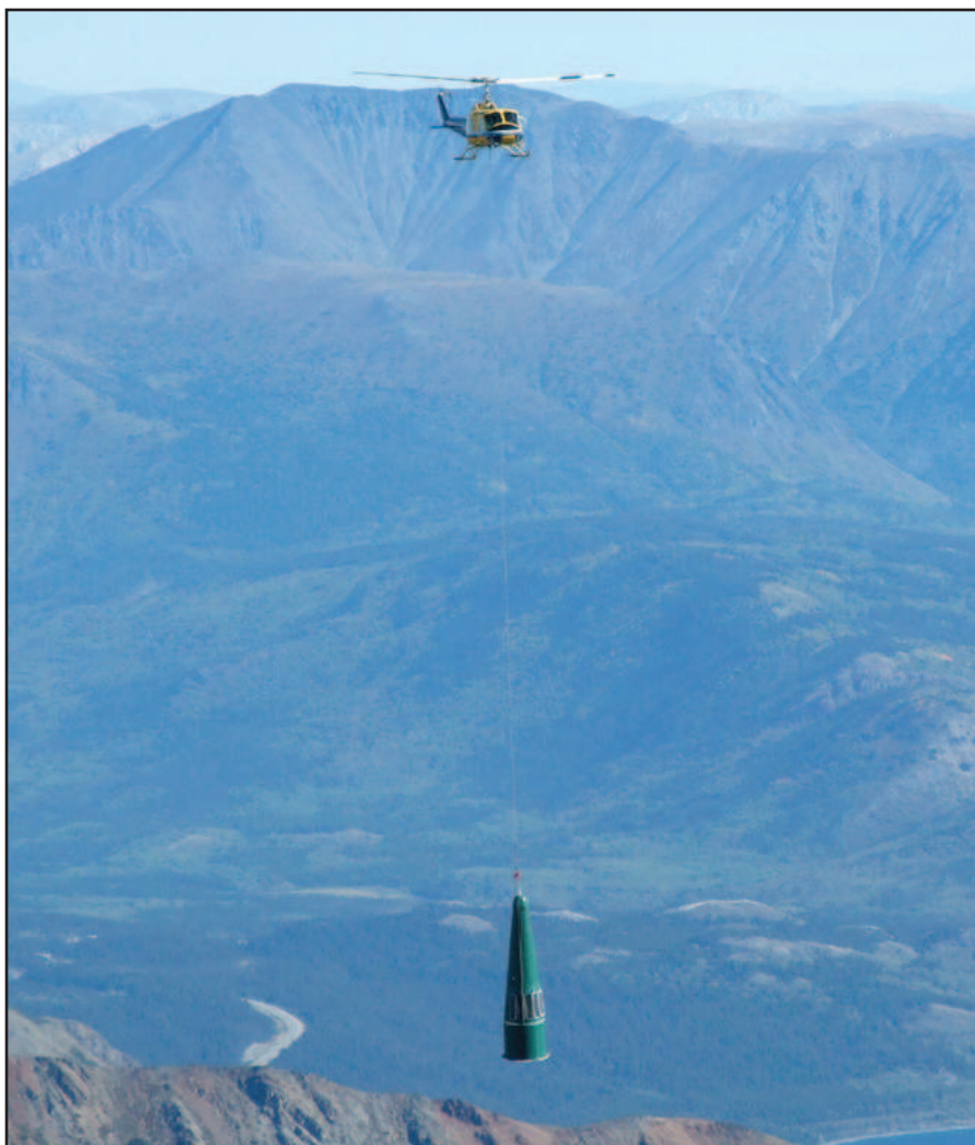
The comshell for Mount Panacea is lifted by a Bell 204 helicpoter.
