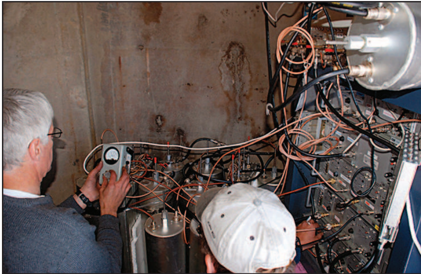
A view inside the lower part of the comshell on Atlin Mountain shows gear at the site, which includes several UHF and VHF transmitters, requiring complex multi-coupling and filtering.
