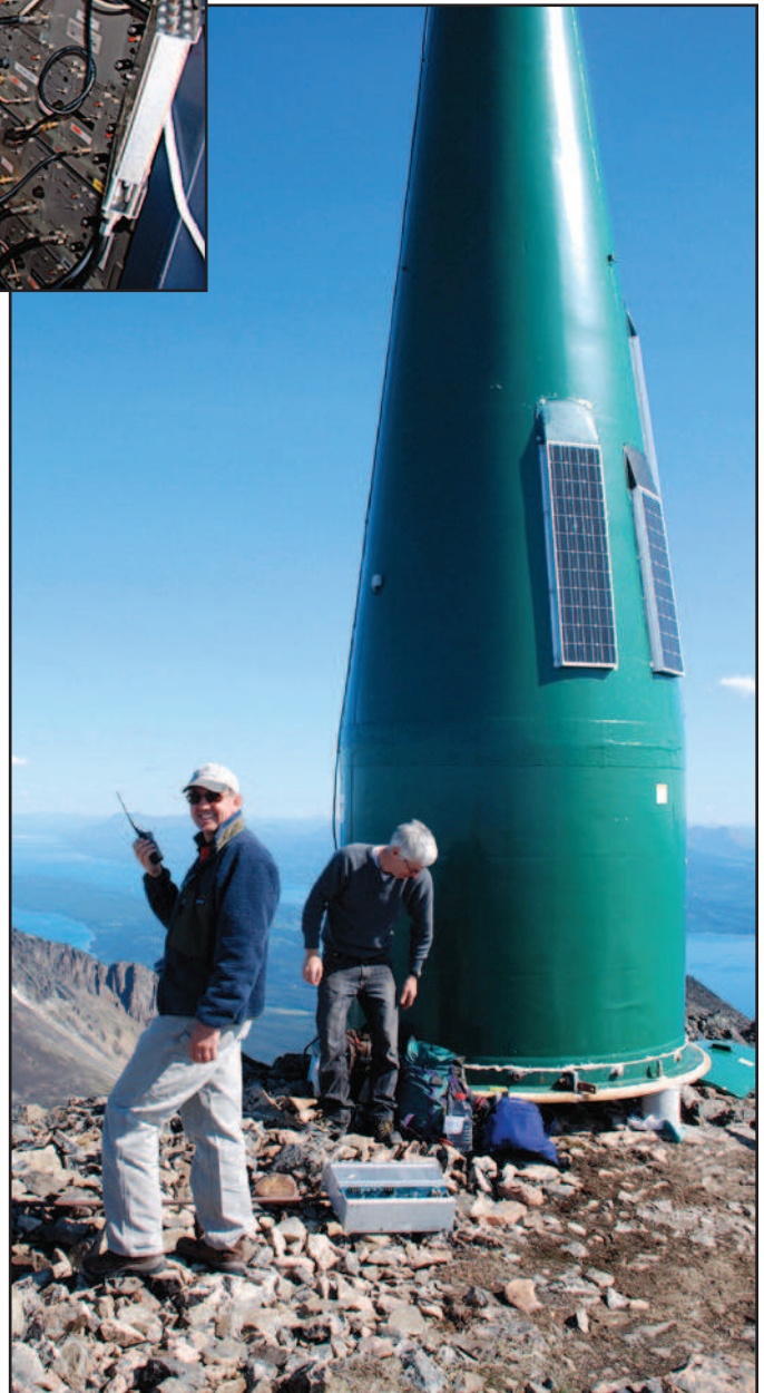
The specially reinforced comshell at the top of Atlin Mountain does not require any guy wiring. All the anchoring is from below with rock anchors and concrete footings. "This was necessary at this site as the mountain drops off quite steeply on three sides of the comshell," VY1SW said. "(You) need to be very careful of footing when stepping out the door as an extra step would take you down a few thousand feet."
